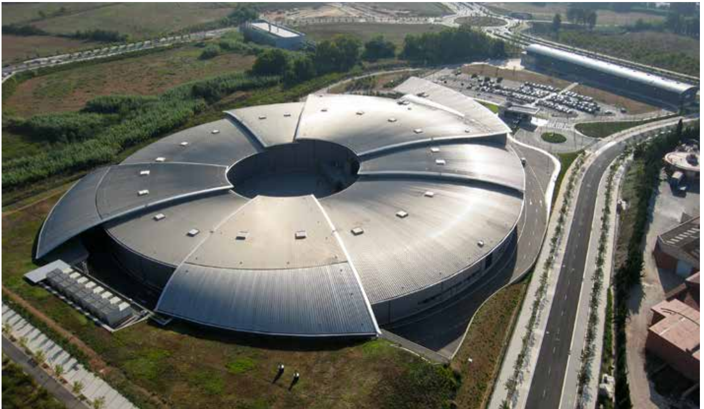
Aerial photograph of the ALBA Sincrotrón complex
